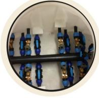
**Main pipe PE100** D40, D63, D90 or D110mm **Outflow PE100**: D32 D40 mm.
